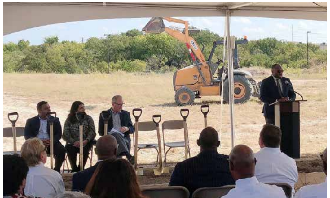
Mayor Steve Mason, alongside partners from Aloft Hotel & TAJ Hospitality, kick-off groundbreaking ceremonies
